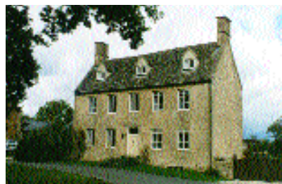
A house of Cotswold Limestone laid in coursed rubble with ashlar quoins, Barton-on-the-Heath, Cotswold Fringe Area
