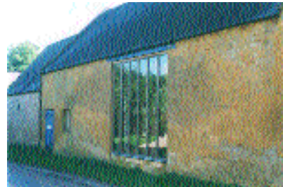
Great Wolford. Appropriate treatment of the midstrey, retaining the full height of the opening.
