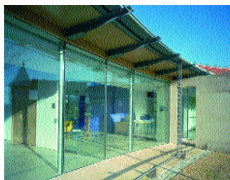
The adaptation of the basic building form is also accomplished by the innovative use of materials. The large areas of glass, galvanised steel and timber extend the traditional palette of brick, clay tile and stone yet, again, the overall effect is a recognisable form that is not at odds with the character of the locality. Photos courtesy of Systems by Design.
