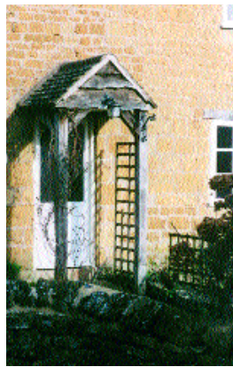
A double pitched canopy on posts, Ilmington, Cotswold Fringe area
