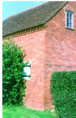
Dentilated brick eaves made up of a projecting stretcher course, alternating projecting headers and a further projecting stretcher course. Priors Marston, Ironstone Uplands area
