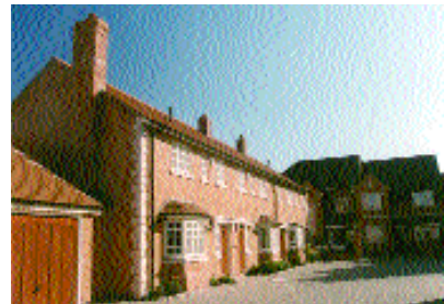
Two different house types used to make the best of a long narrow plot in a new development off High Street, Henley.
