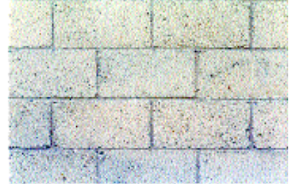
Concrete block wall
