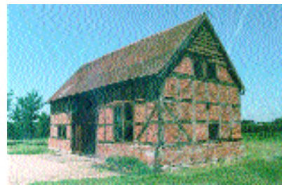
Converted barn in Moreton Bagot, Arden area. Note that the openings are contained within the timber frame structure
