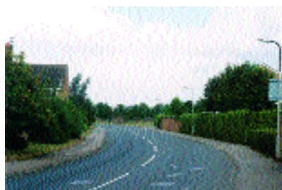
A result of cul-de-sac development: a blank, inhospitable estate distributor road
