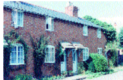
Cottages with windows set just below the top plate in Welford-on-Avon, Avon Valley area. The casement windows shown are flush closing as opposed to 'storm proof'
