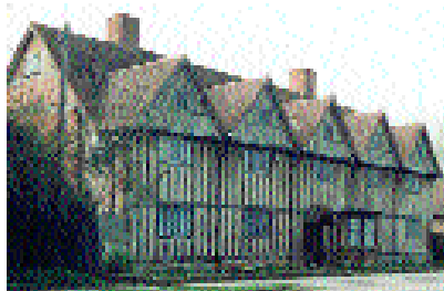
A close studded timber framed house with rendered infill panels in Long Itchington, Feldon area
