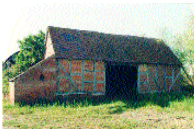
Timber framed barn with brick infill, Haselor, Arden area
