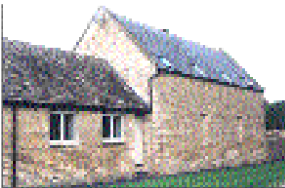
Sensitive conversion in Long Compton with simple, restrained flush closing casement windows and rooflights set flush with the roof.
