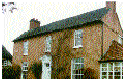
A house with walls built in Flemish bond with buff headers, Wellesbourne, Avon Valley area. The windows have flat brick arch heads and stone cills. Note that the cills are slightly wider than the window opening.
