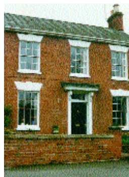
Render used to create the effect of stone lintels in Wellesbourne, Avon Valley area. The windows have stone cills and sliding sash frames.
