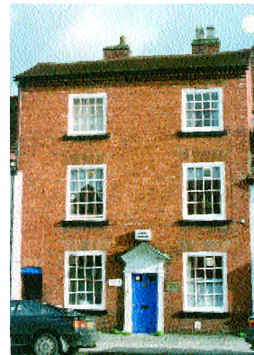
A brick house with rubbed brick flat arch window heads in Henley-in-Arden, Arden area
